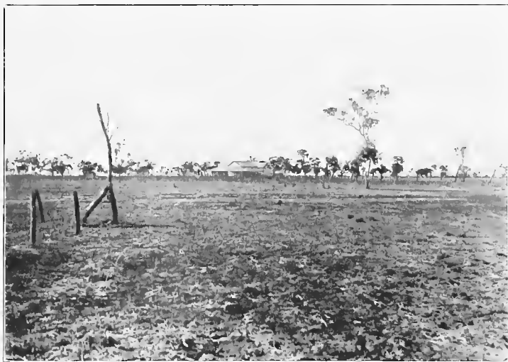
Fig. 344. POLICE QUARTERS, BORROLOOLA.
